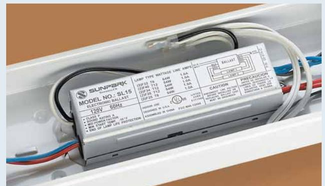
You'll find the noise rating printed on the ballast as well. A rating system of A, B, or C is most commonly used, with "A" offering the quietest operation.
